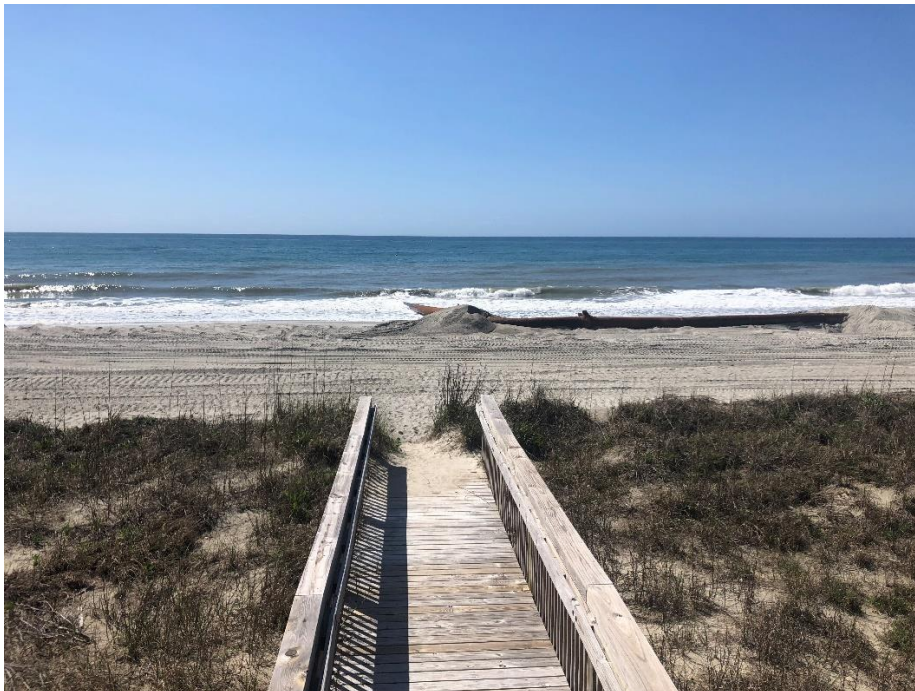
Figure 1. A typical wooden structural accessway.
